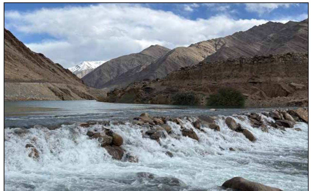
Photo Caption: Rock Check Dam over the River Indus at Upshi in Leh district.
