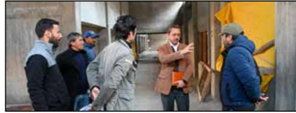
Administrator Municipal Committee Kargil and Joint Director Information UT Ladakh, Imteaz Kacho inspecting various ongoing developmental works.
