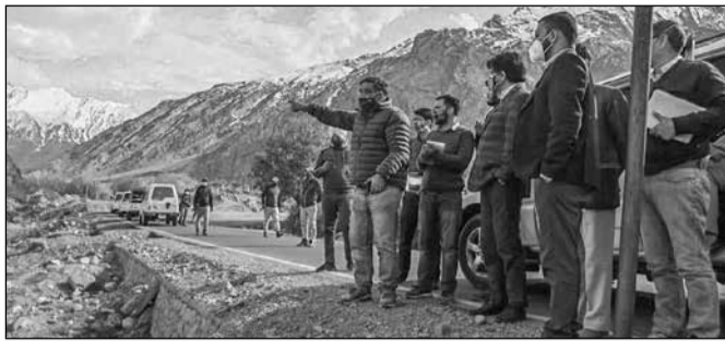
CEC, Hill Council, Kargil, Feroz Ahmed Khan along with DC, Kargil, Santosh Sukhadeve and other officials taking stock of the ongoing widening and construction works on the Kargil Zanskar Road NH-301.
