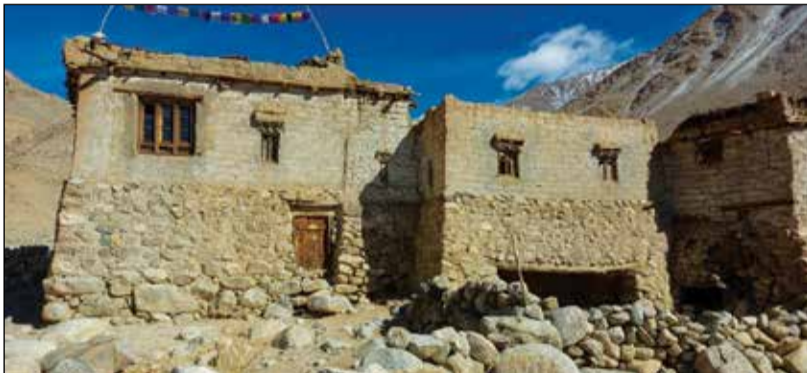
Old abandoned house of Kulum village.
