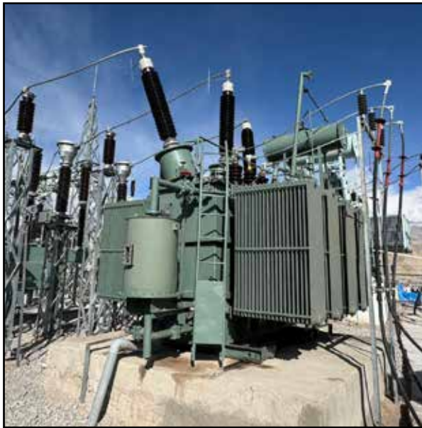
Photo Caption: 10 MVA power transformer installed to augment the capacity of the Chuchot Substation.
